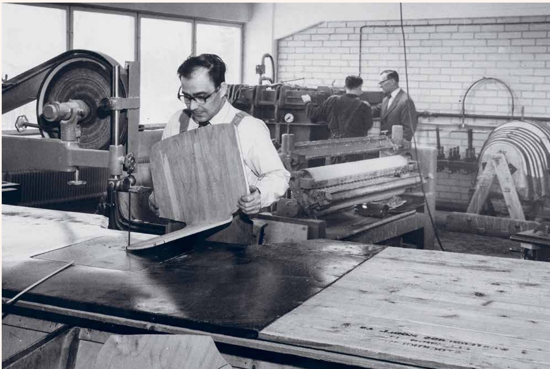
Snapshot from the Puunveisto Oy workshop in the 1950s. In the background, designer Hiort af Ornäs looks on as the frame of a Siesta lounge chair is being moulded.
